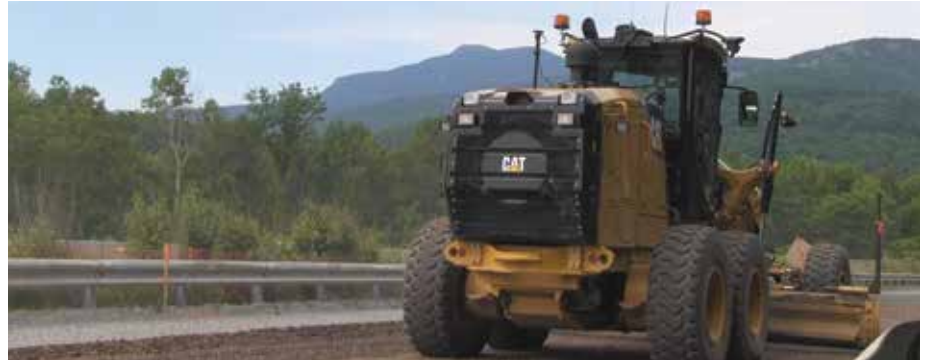
WATERBURY/BOLTON. Reclaiming US 2 eliminated on-going maintenance issues by removing narrow concrete slabs that had been under the roadway for more than 50 years.
