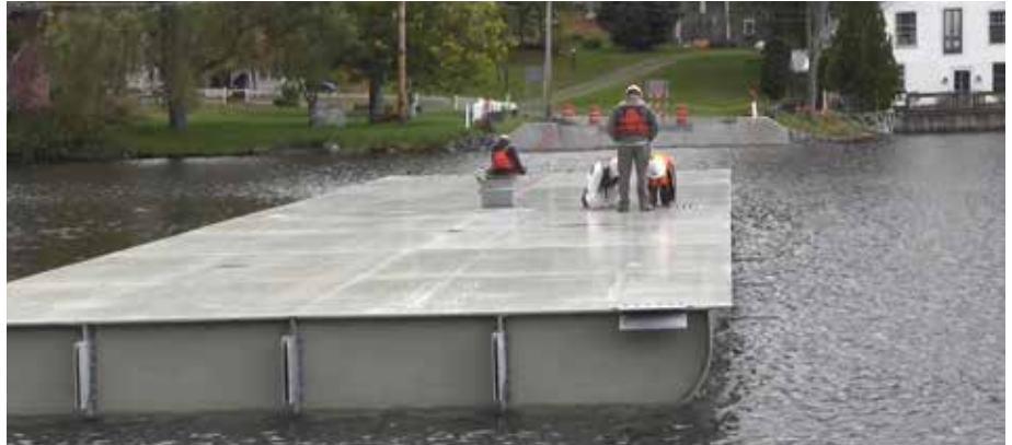
BROOKFIELD. Moving a new section of the “Floating Bridge” into place.
