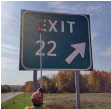
HIGHGATE. Testing a sign on I-89 with a retroreflectometer.
