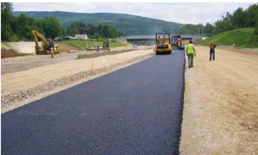
BENNINGTON. VT 279. An example of engineered pavement.
