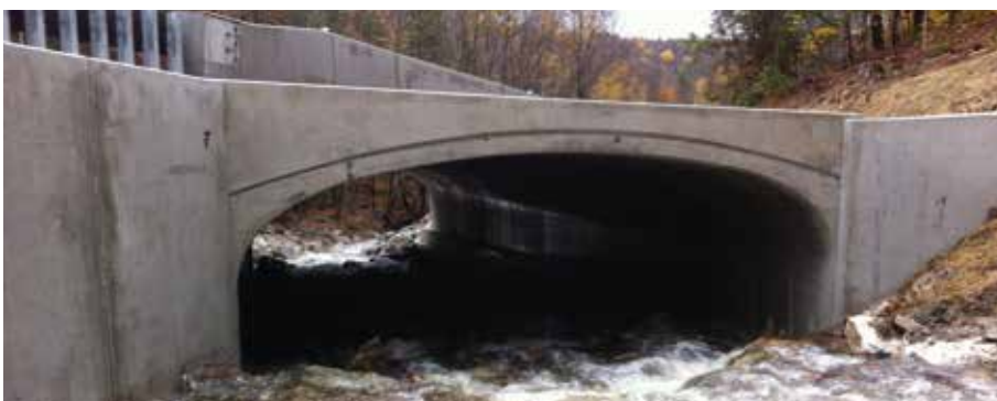
ROCHESTER. Bridge 13 is designed with aquatic organism passage and storm resilience in mind.
