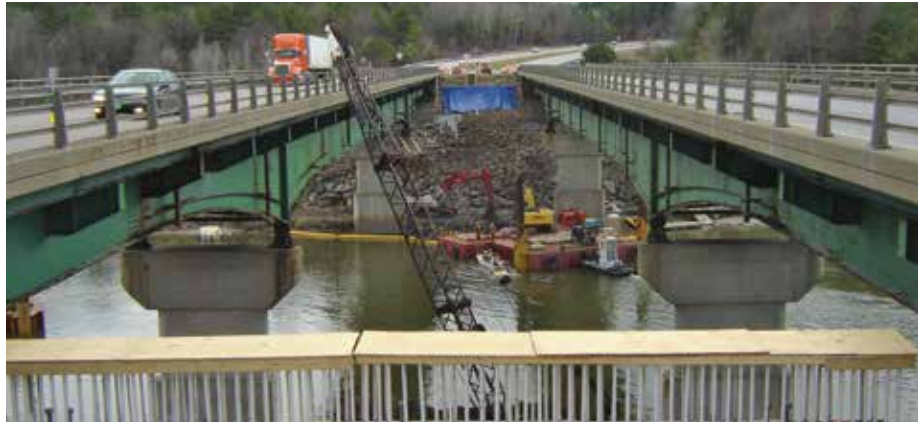
MILTON. Constructing a new bridge over the Lamoille River on I-89 between existing spans.
