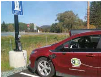
HARTLAND. Newly upgraded park and ride includes Level 1 Electric Vehicle charging.
