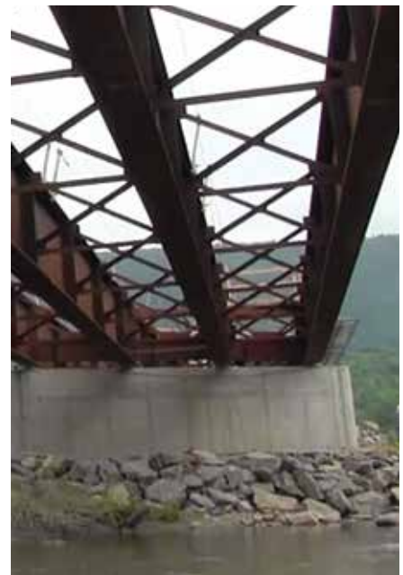
BRISTOL, VT. 116 Replacement project.
