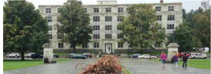
MONTPELIER. DMV main office.
