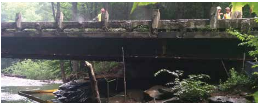
WARREN. VT 100 Bridge before replacement.
