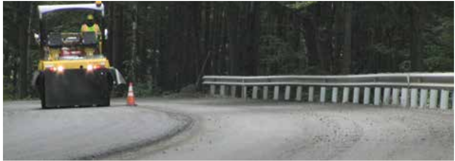
STOCKBRIDGE / BETHEL. Paving project.
