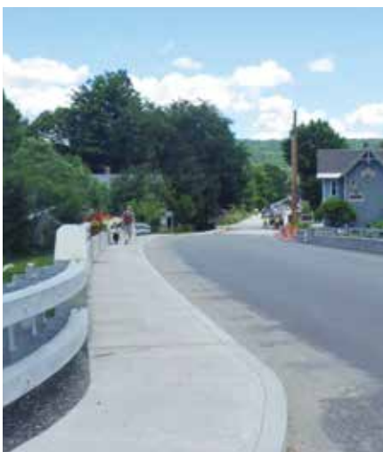
JAMAICA. This bridge on VT 30 was developed and designed in 11 months through the ABP.
