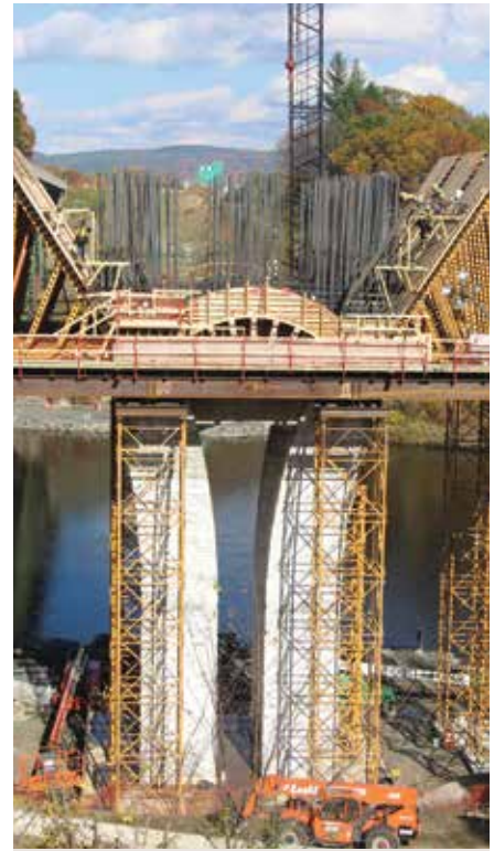
BRATTLEBORO. Erecting the pier of the new "Bridge to Nature" on I-91.
